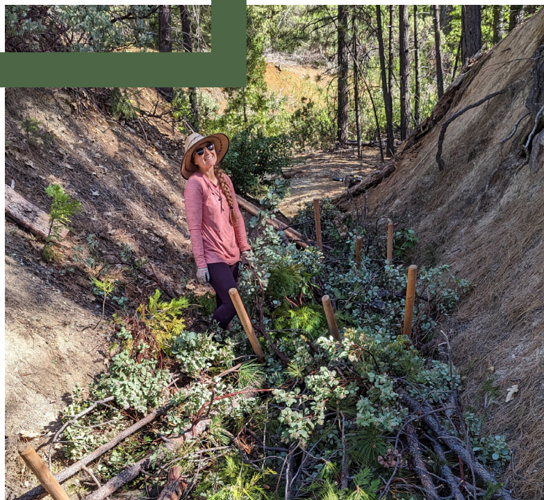
Photo: Work crew member installing a post-assisted log structure at Grizzly Creek.
